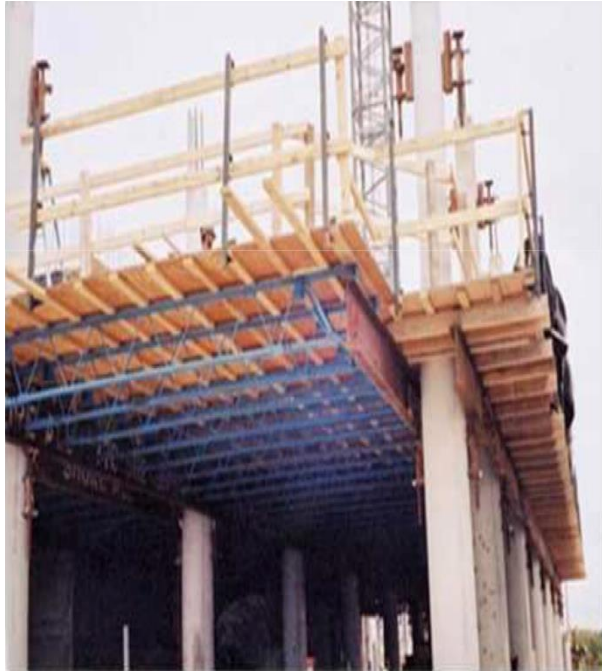
Figure 17: The column mounted shoring system
