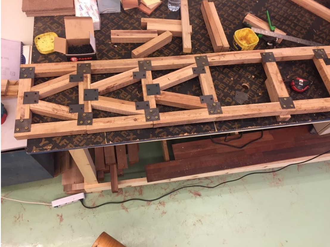
Figure 71: Connecting the inner diagonals of the truss
