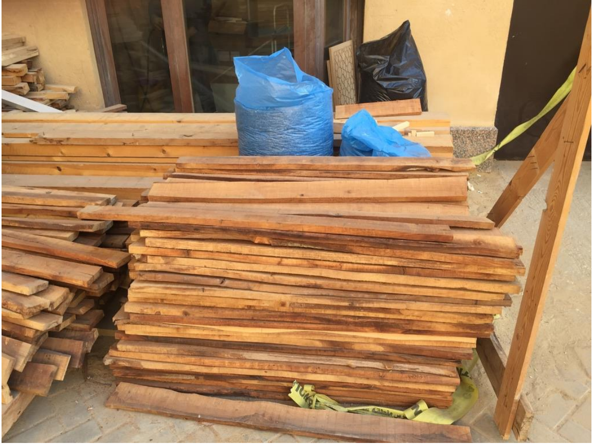
Figure 66: The procurement of the wood used in manufacturing the trusses
